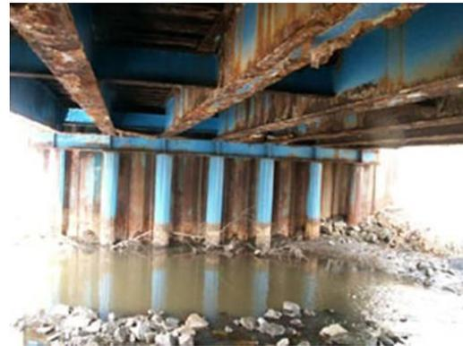
**Figure 2. Corroded steel bridge girders**
