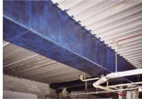
**Figure 4. Picture showing beam retrofit using CFRP**
